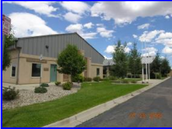
West side of U-shaped building at 4950 Geiger with 800 SF Offices in front.
