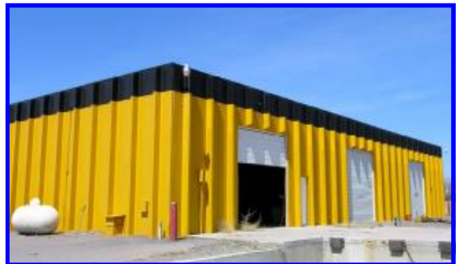
Rear view, propane tank, and truck dock
