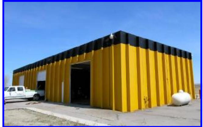
Southwest Corner of building—12' Doors
