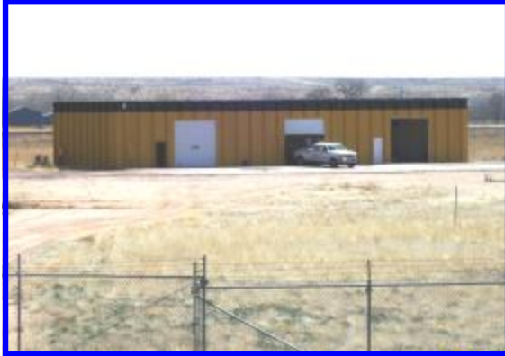
View looking east from Front Gate
