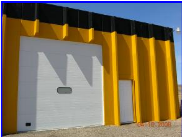
Rear Overhead and people door
