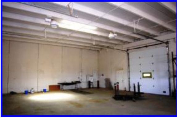
North Side—Interior of 105' x 40' Building
